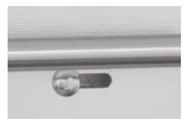
Adjustable air inlet integrated in the door
